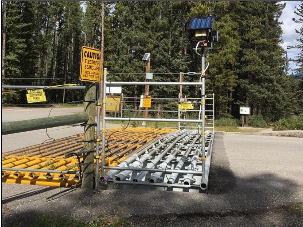
Figure 6. Electrified cattle guard at Lake Louise campground. Photo by J. Marley.
