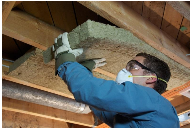
Figure 13: Using of insulation material in modern building [19]
